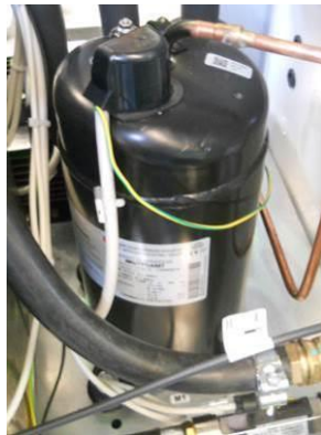
Picture 21 – Compressor placement
